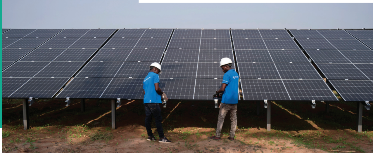
Solar technicians installing panels at a mini-grid site Image Courtesy: EmekeObanor/Ashden/Sosai
